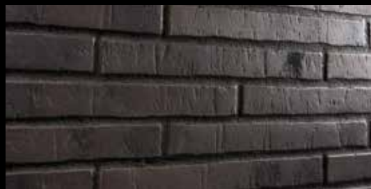
The finished joint pattern after slurry treatment.
