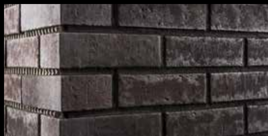
The finished joint pattern. Full masonry stretches are grouted at one go.
