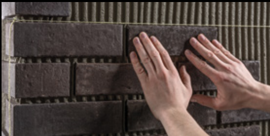
Use a string to plumb the clinker area. The clinker slips are pressed into the adhesive bed.
