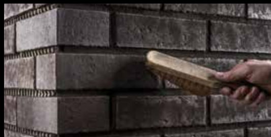
Sweeping out the joint gives it a corresponding structure.
