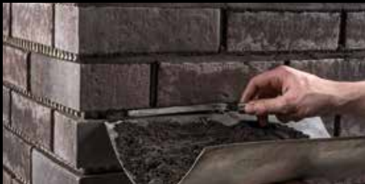
Grouting using pointing trowel and metal float along the horizontal.
