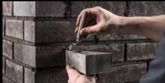
The vertical joints can be finished more easily with a smaller pointing trowel.
