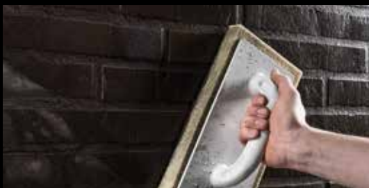
The excess grout is washed off diagonally using a plaster float with a sponge or foam pad.
