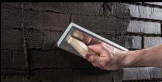
With the slurry method, the joints are filled diagonally with the grouting or plaster float. Walls should be worked from top to bottom.
