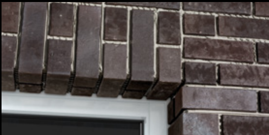
Window lintel perfectly replicated with angles.
