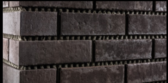
The finished surface. Grouting can be done after the appropriate drying time.
