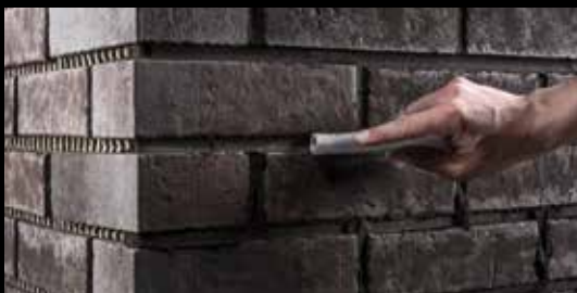
Jointing with a trowel allows you to create different looks.
